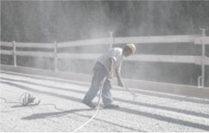
Clean the holes by brushing and blowing out with compressed air using the appropriate Hilti accessories.
