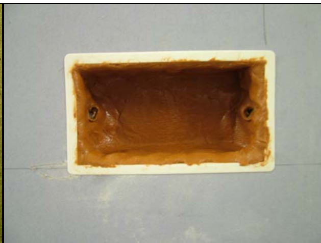
Photograph 4. Hilti Putty Pad fitted into wall box
