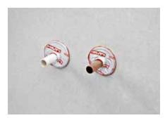
MV: Electric Power Conduits: Plastic / Metal
